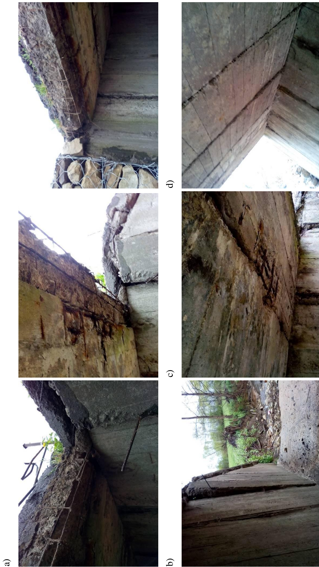
Fig. 3. Typical defects of reinforced concrete structures of the bridge:
