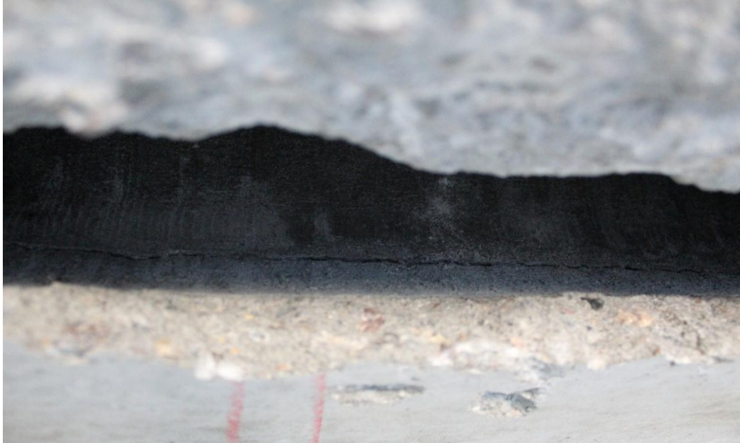
Fig. 4. A crack that appeared in the rib between the cavities
