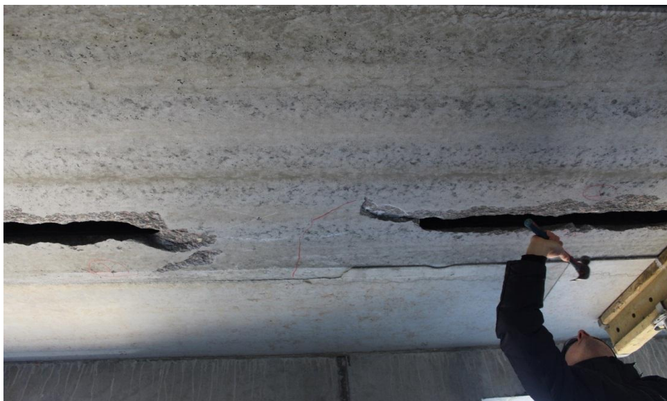
Fig. 5. Contours of damage after reflection of exfoliated surface layers
