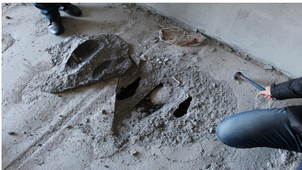
Fig. 1. Destruction in the upper part of the slab
