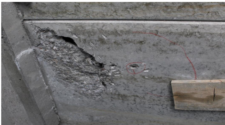
Fig. 2. Destruction in the lower part of the slab
