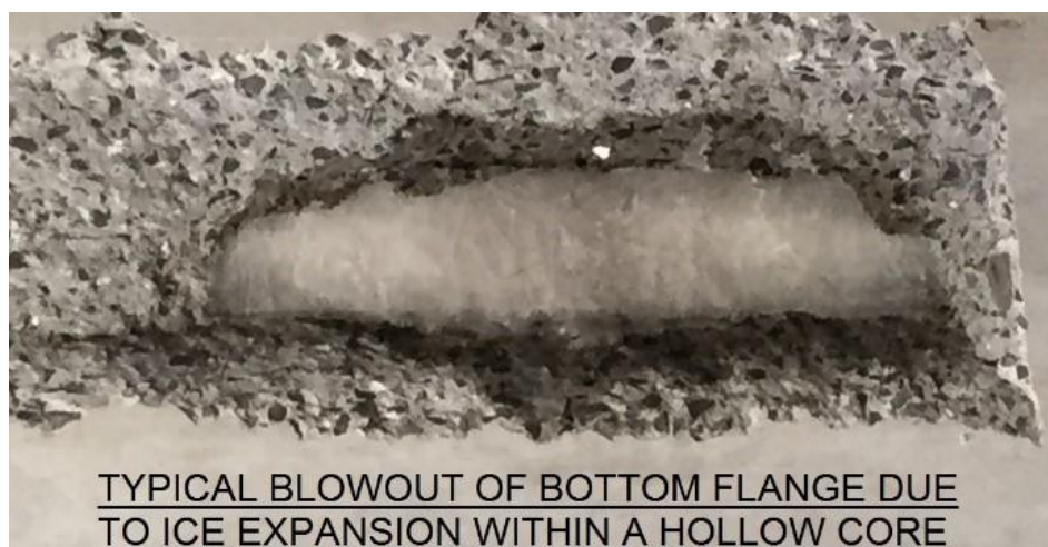
Fig. 3. Typical chipping of the lower shelf of the plate due to the expansion of the ice the USA, Maryland
