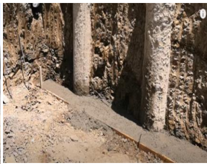
e – concrete foundation is performed
