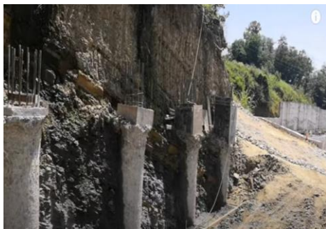
d – general view of piles
