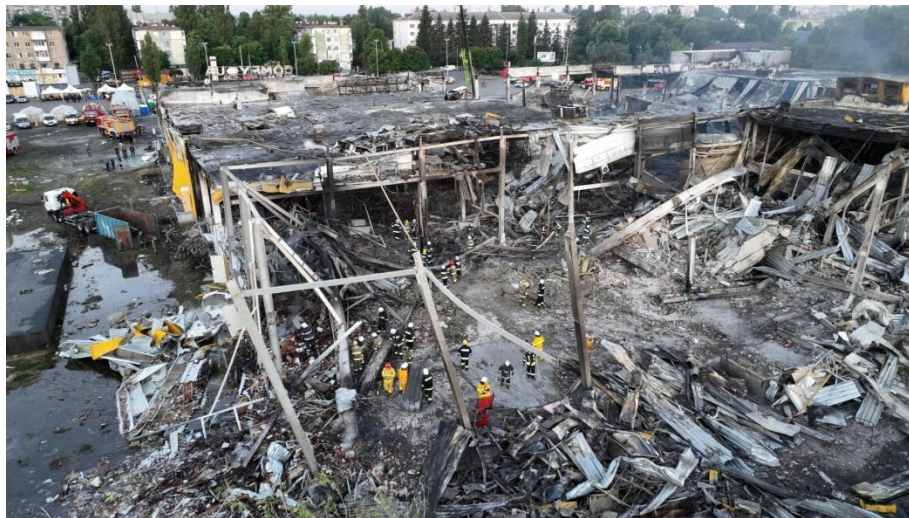
Fig. 2. The result of building progressive collapse from a missile strike and fire in the shopping center in Kremenchug
