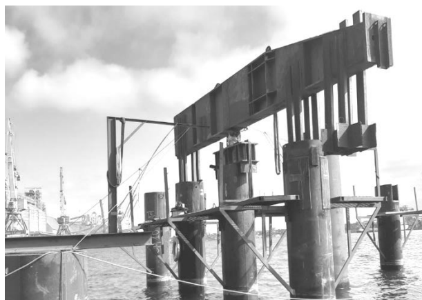
Fig. 1. Test bench for testing the piles with static loads
