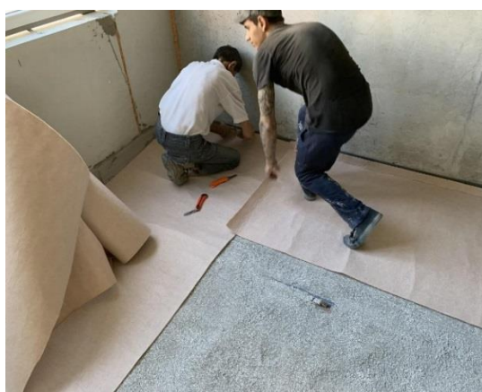
Fig. 3. Laying material "Akuflex"
