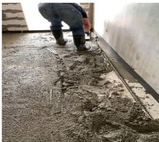
Fig. 2. The installation of "Izolkap"
