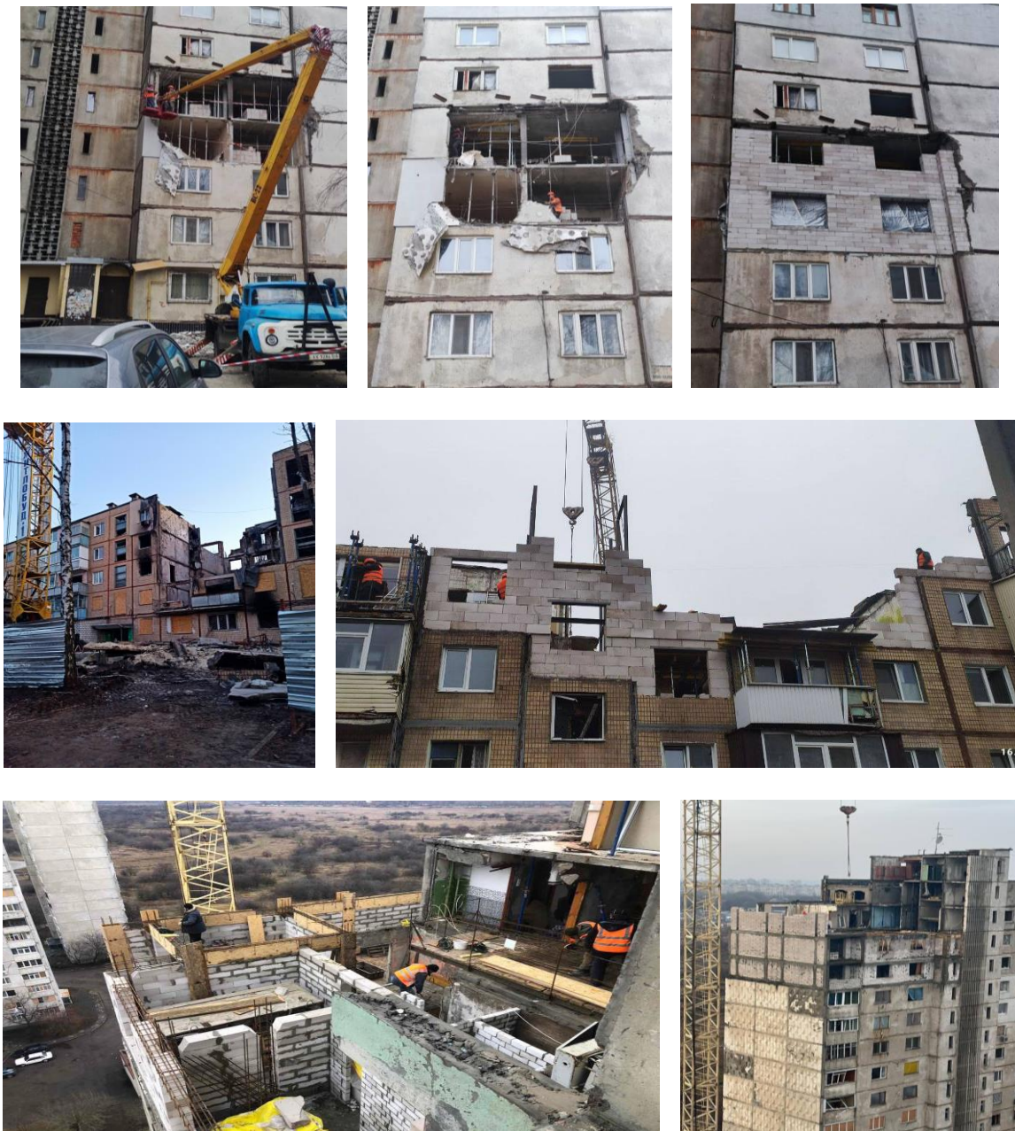
Fig. 2. Restoration of damaged multi-storey residential buildings in the city of Kharkiv
