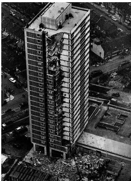
Fig. 1. The collapse of the Ronan Point residential building in London, Great Britain, 1968
