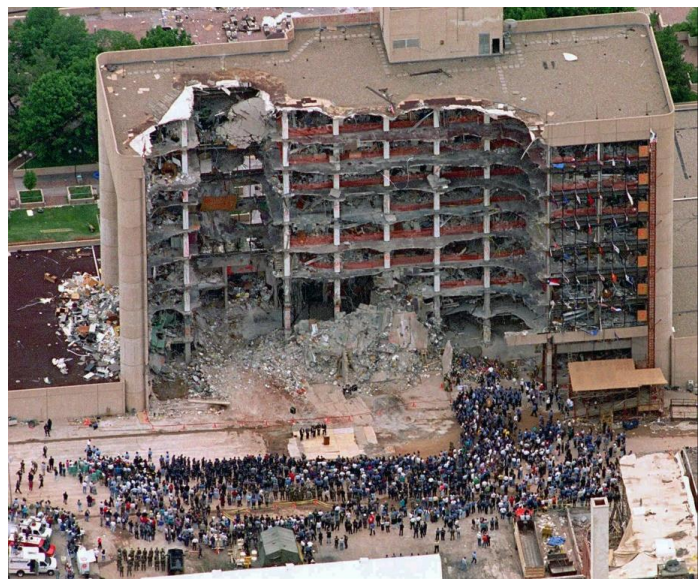
Fig. 2. Collapse of the Alfred P. Murrah Federal Building in Oklahoma City, USA, 1995
