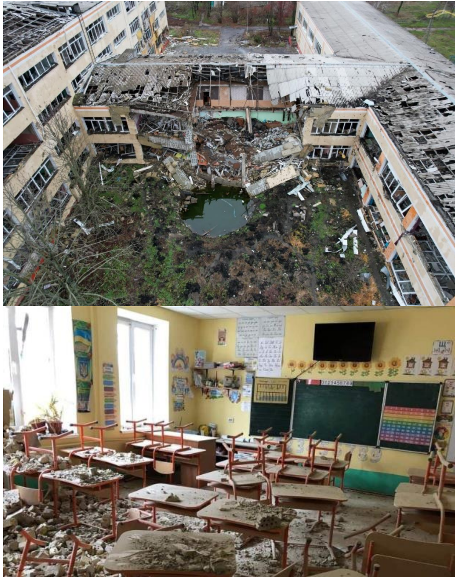
Fig. 1. Damaged educational facility
