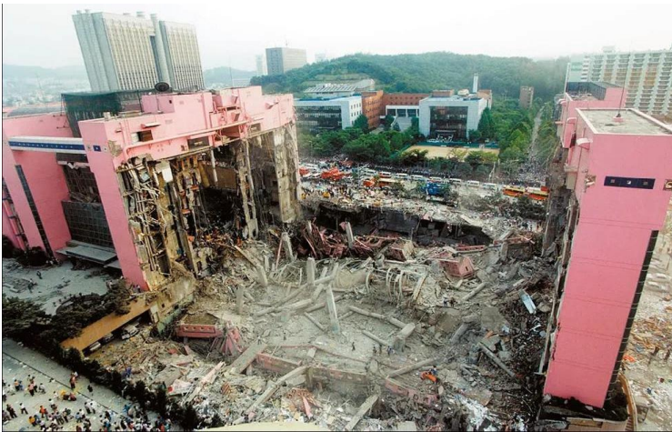
Fig. 3. Collapse of the Sampoong shopping center in Seoul, South Korea, 1995
