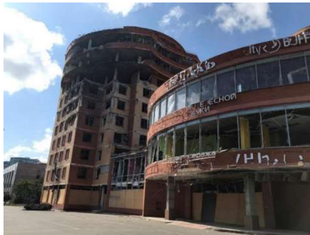
Fig. 1. General appearance of the facade of the building
