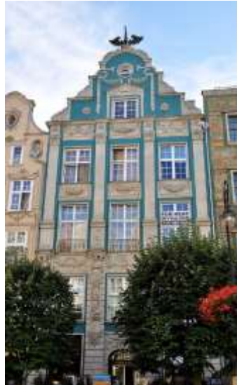
Fig. 2. Building at the address: Długi Targ str. 20 (photo by Aleksandra Wolska)
