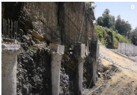
d – general view of piles
