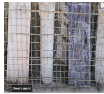
f – installation of internal formwork and reinforcing frame
