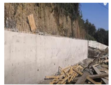
i – general view of the retaining wall
