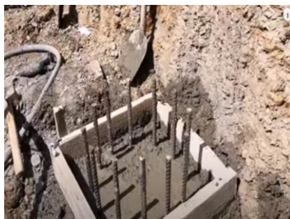
b – concreting of a pile
