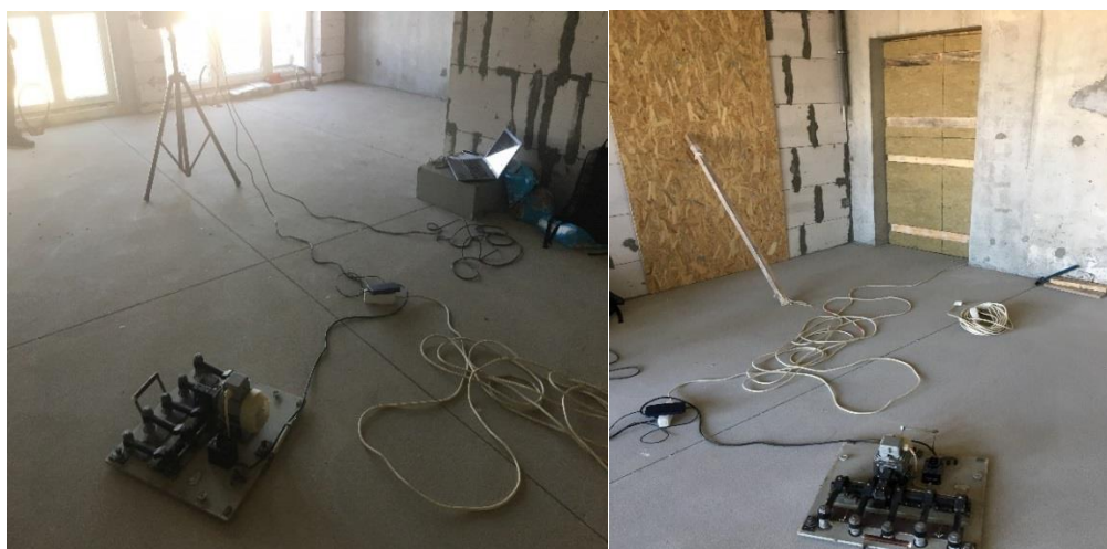
Fig. 5. Measurement of impact noise insulation
